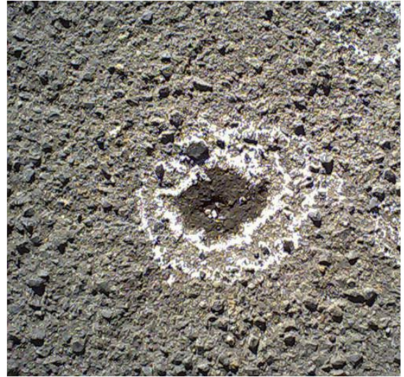
Figure 8: Impact of salinity on road base
