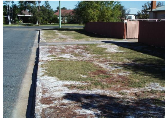
Figure 8: Impact of salinity on road base
